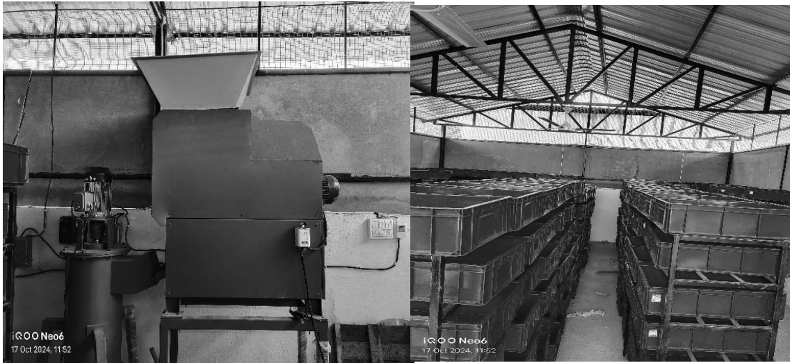
Figure 1- Installation of Grinding machine
