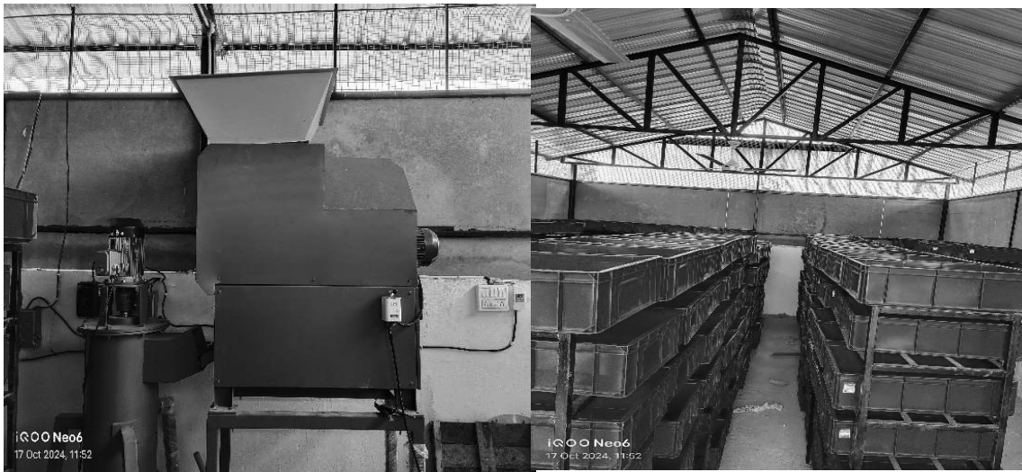
Figure 1- Installation of Grinding machine
